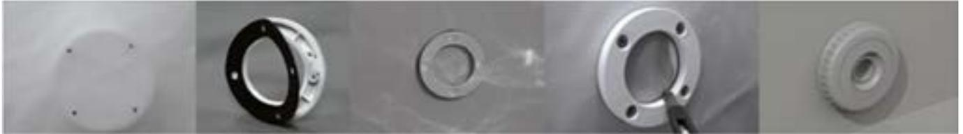
Figure 29 – Installing the return fitting flange
