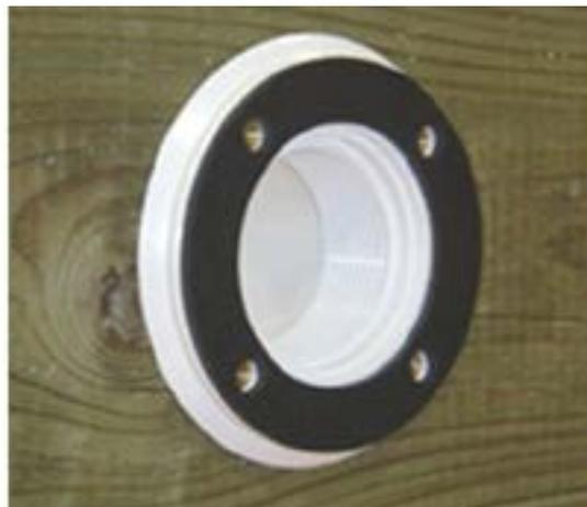
Figure 24 – Mounting the return fitting body and gasket
