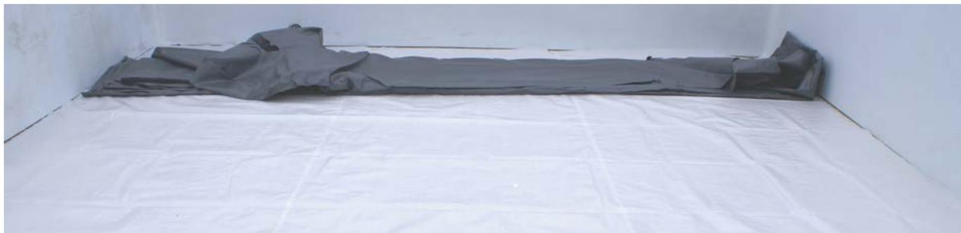
Figure 27 – Unfolding the liner
