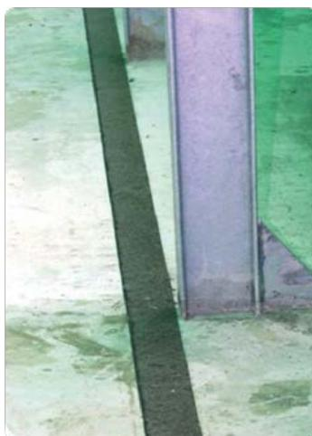
Figure 7 – Laying the bituminous strips
