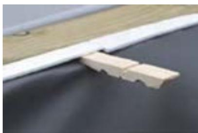
Block the liner in position with half-pegs (not supplied) as you progress around the pool, pay particular attention to the corners *Figure 28*).
