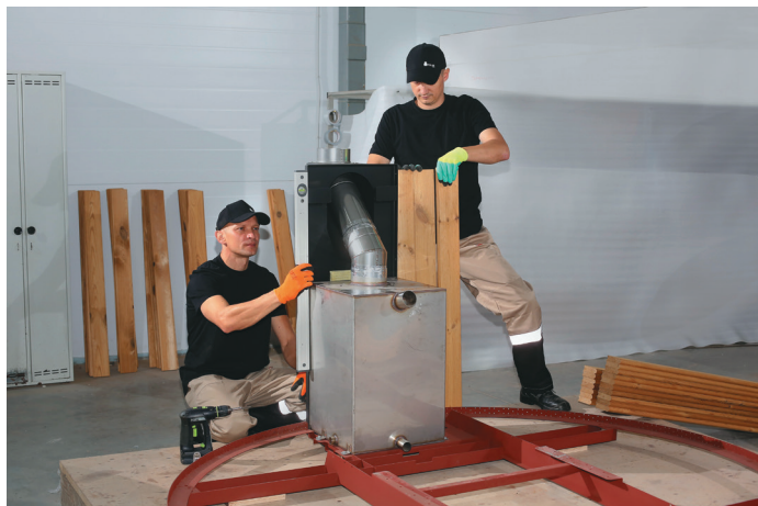
Installation of the furnace on the metal frame.
