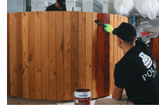
Varnishing the thermal wood with a protective coating
